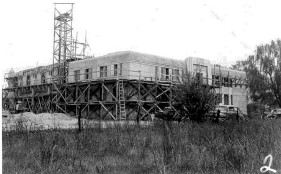
St. Matthews Armory construction. 1940-11-23 - 1942-7-16
